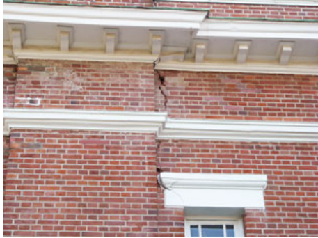
Cracks in the main building
