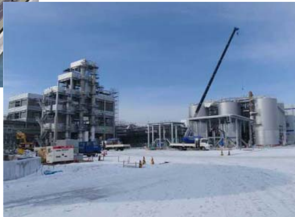
Construction site (at the beginning of February)
